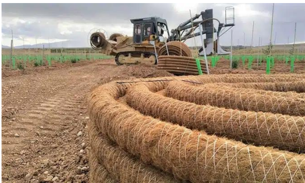
Horizontal French drain system
