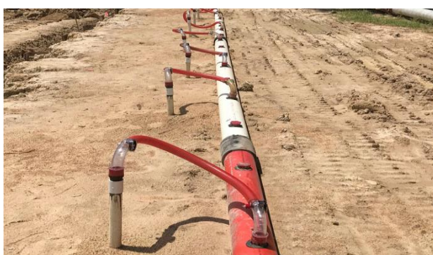
Vertical well-point system
