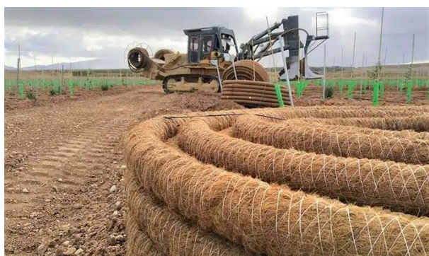
Horizontal French drain system
